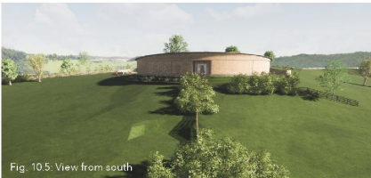
Fig. 10.5. View from south
