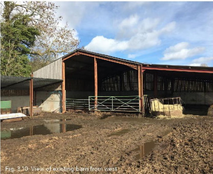
Fig. 3.10 View of existing barn from west
