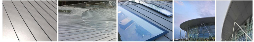
Fig. 9.8. Examples of zinc roofs
